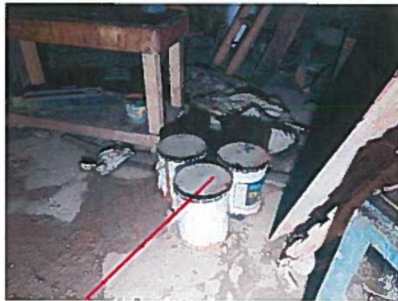
Miscellaneous paints and chemicals noted within the structure.
