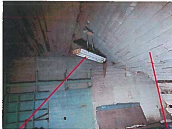
Tubes in Fluorescent light fixtures contain Mercury. Note falling ceiling.
