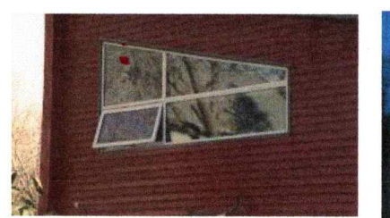
Building 2 homes on 1 property: A look ... globalnews.ca
